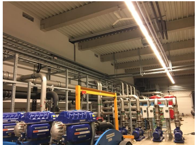
Figure 3: XHM pump house installation.
